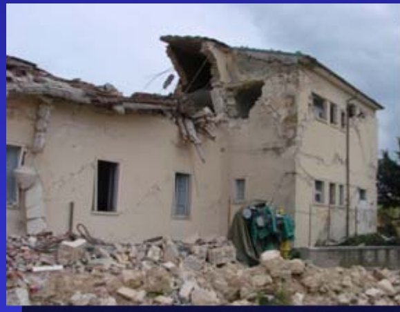
Damage level 4: serious structural
