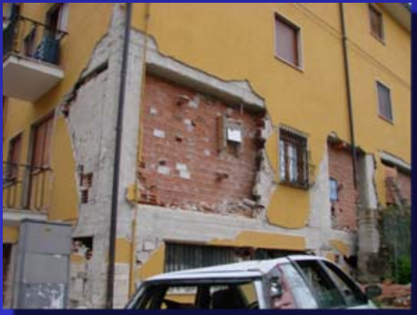
Damage level 3: architectural
