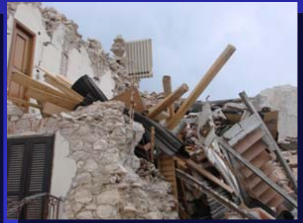
Damage level 5: collapse
