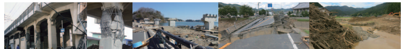
Field surveys on lifeline damages
